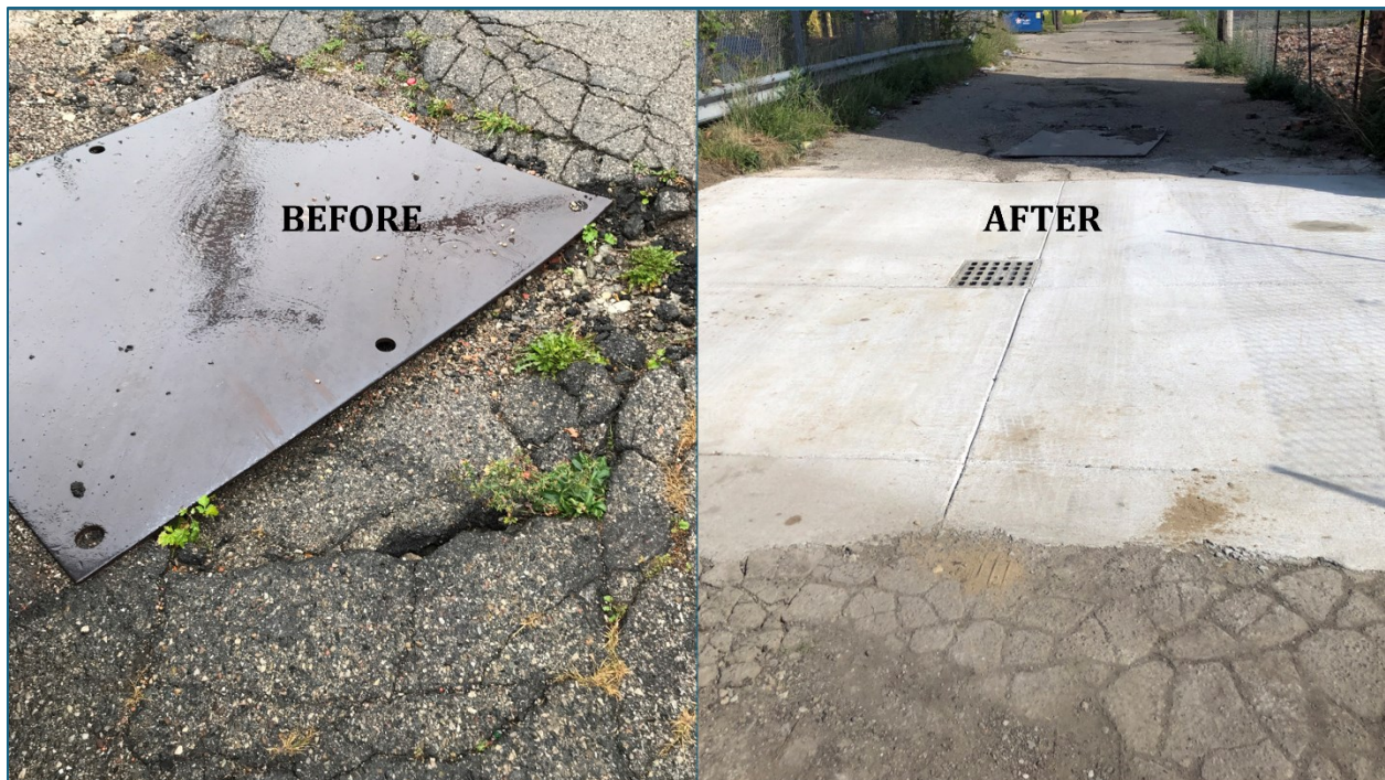
Figure 47: Example of Large Sinkhole Repair Before & After
