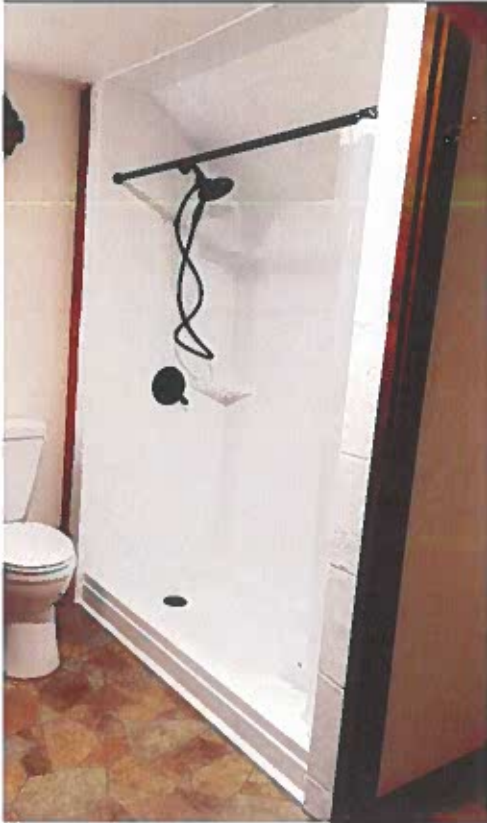
Typical shower insert install. No door. Small lip on drainage tray. Possibly grab bars and handhead shower heads.
