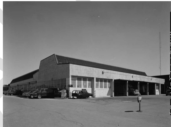
FIGURE 2. Chrysler Center, Plant No. 4
