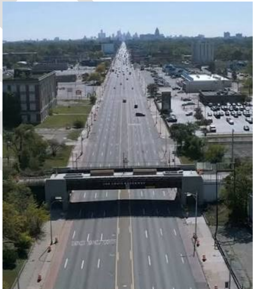
FIGURE 1. Joe Louis Greenway Pedestrian Bridge at Woodward
