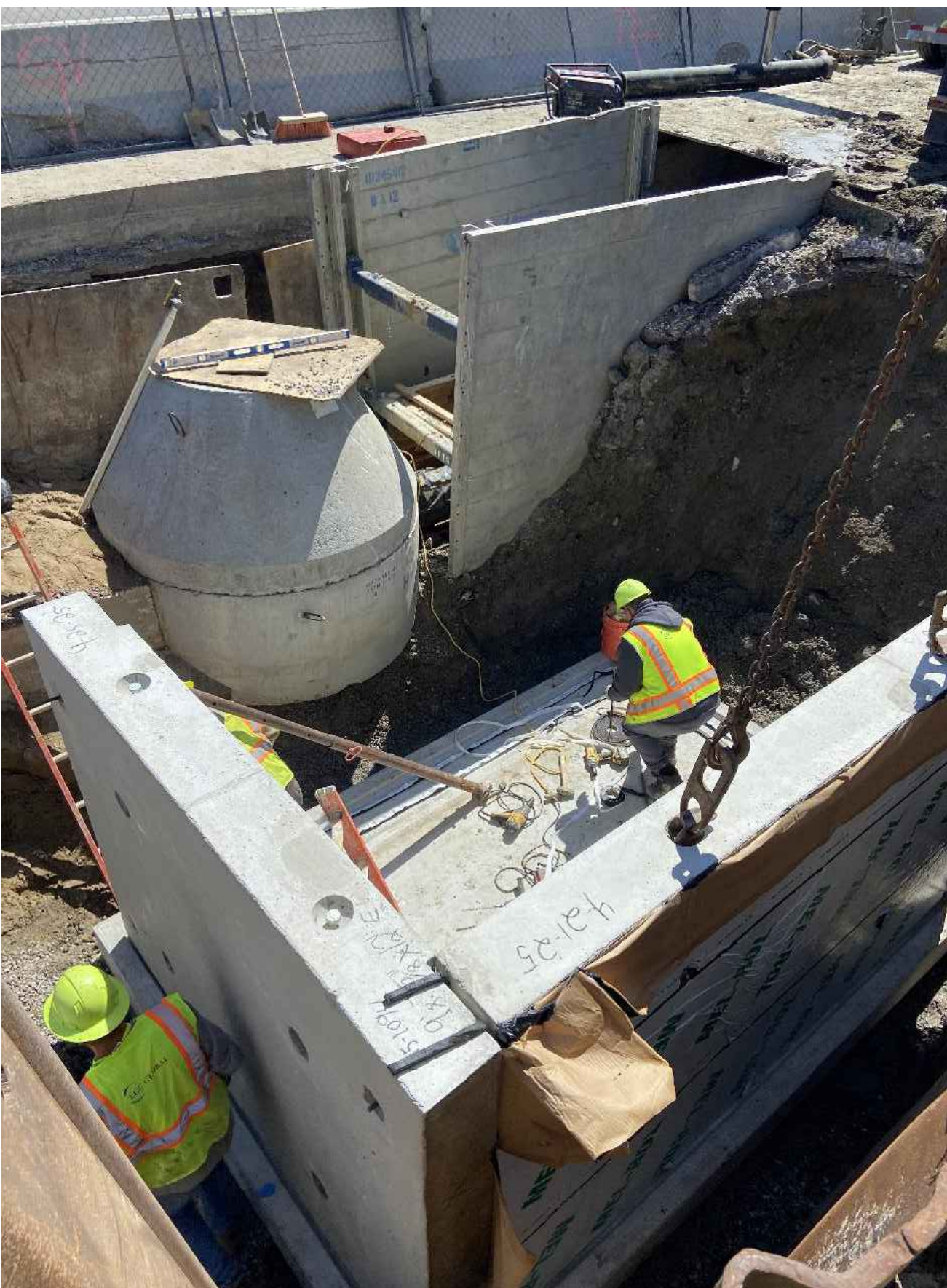
MASTER METER HP-07 VAULT AND BYPASS VALVE CONSTRUCTION
