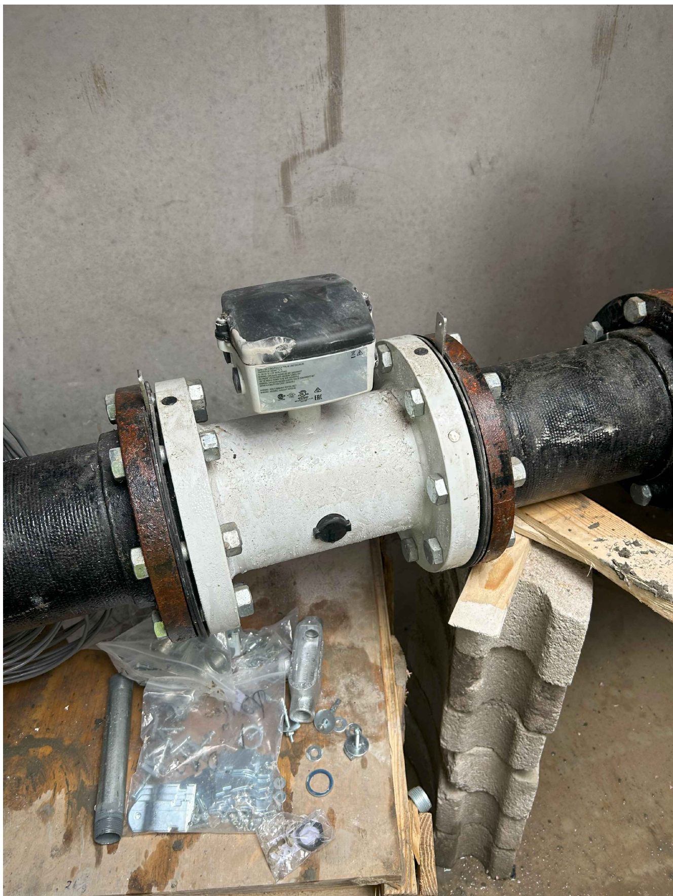
INSIDE VAULT: MASTER METER APPARATUS
