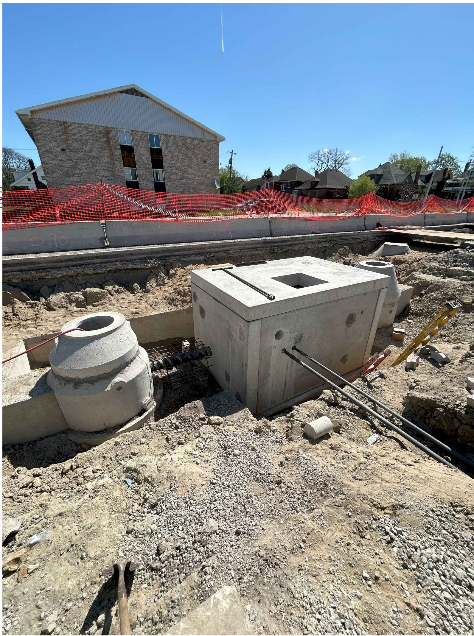
MASTER METER HP-07 VAULT AND GATE VALVE CONSTRUCTION
