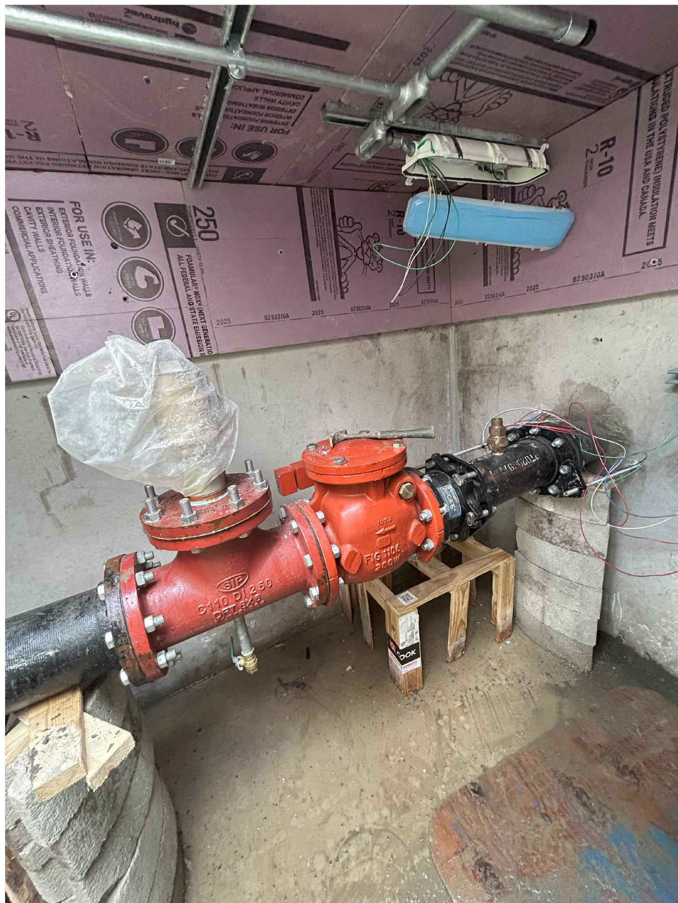
INSIDE VAULT: METER AND CHECK VALVE CONFIGURATION
